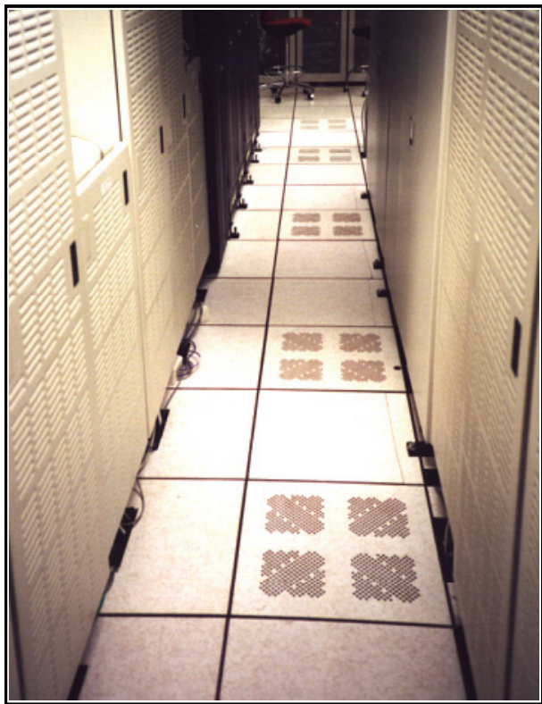
Figure 3. These misplaced perforated tiles and less obvious unmanaged cable openings are allowing valuable cold air to escape. Forty-five percent of the capacity of a 20-ton cooling unit is being wasted in this picture.
